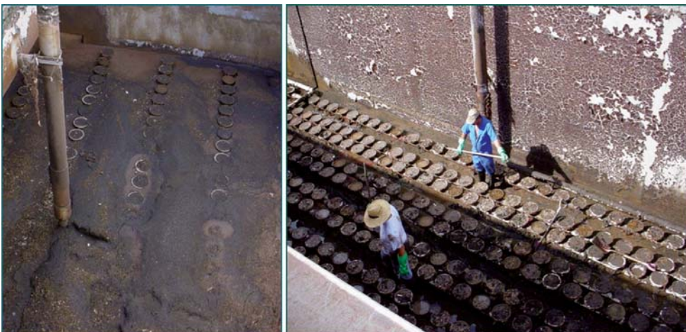
Figure 1. Grit deposition in fine bubble aeration basin.
